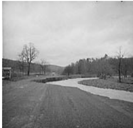
Road washed out by a flood in West Virginia. Source: A. Rothstein, Farm Security Administration.
